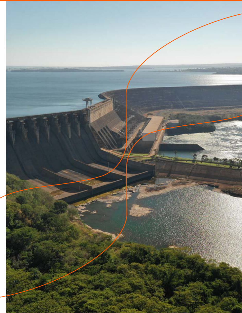
The São Simão power plant, on the border between Minas Gerais and Goiás states
